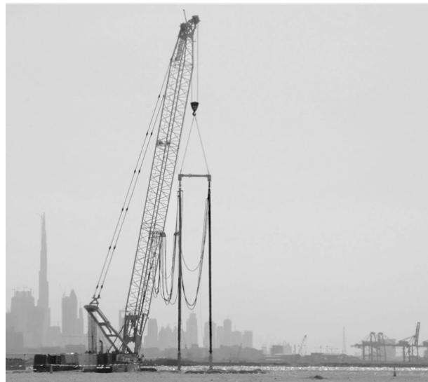
Figure 10. Tandem Vibro Compaction, Dubai.
