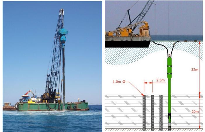
Figure 13. Submersible rig with water pump
