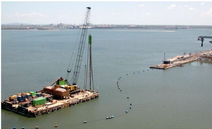
Figure 5. Stone columns installation at Richard Bay
