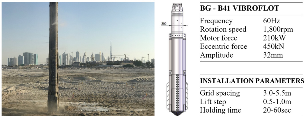
Figure 1. Typical equipment and installation parameters for vibro compaction works.
