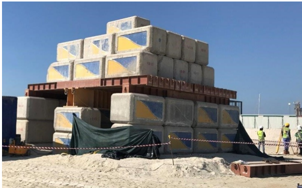
Figure 3. Large scale plate load test.
